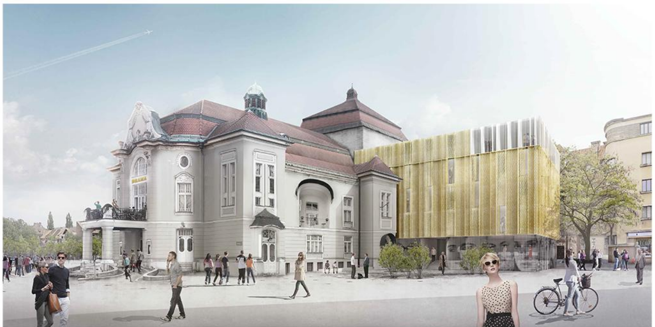
ZAHODNO KRILLO JE NAMENJENO DRAMSKIM DELAVCEM Z VHODOM ZA ZAPOSLENE IN SE V ZGORNJEM VOGALU ZAKLJUČUJE S PROSTOROM JEDILNICE Z RAZGLEDOM PROTI CANKARJEVOM DOMU. EAWEST WING IS DESIGNATED TO DRAMA EMPLOYEES, WITH THEIR ENTRANCE AND DINING ROOM ON TOP FLOOR WITH THE VIEW TOWARDS NATIONAL CULTURAL CENTRE CANKARJEV DOM.
