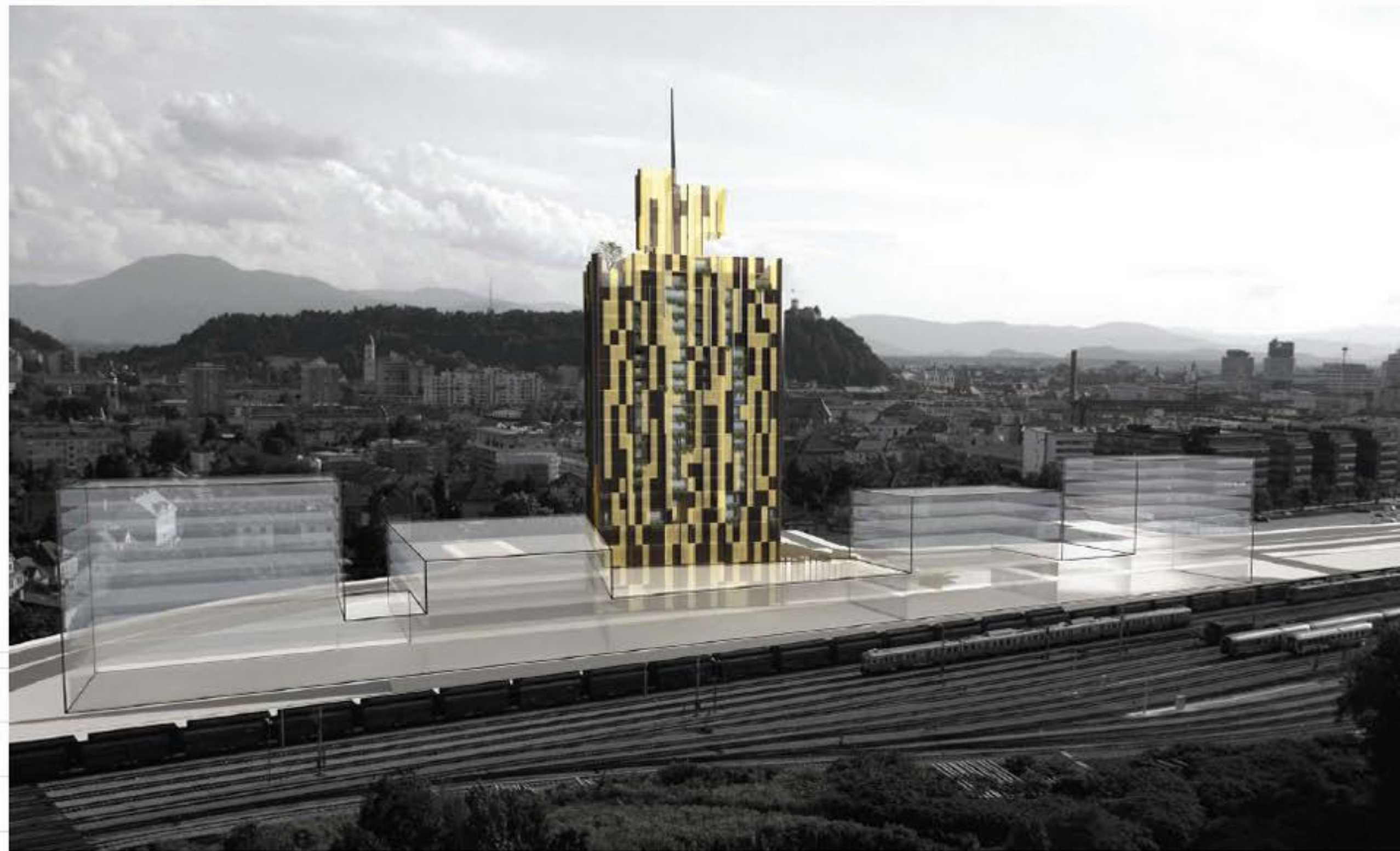
POGLED S SEVERA
