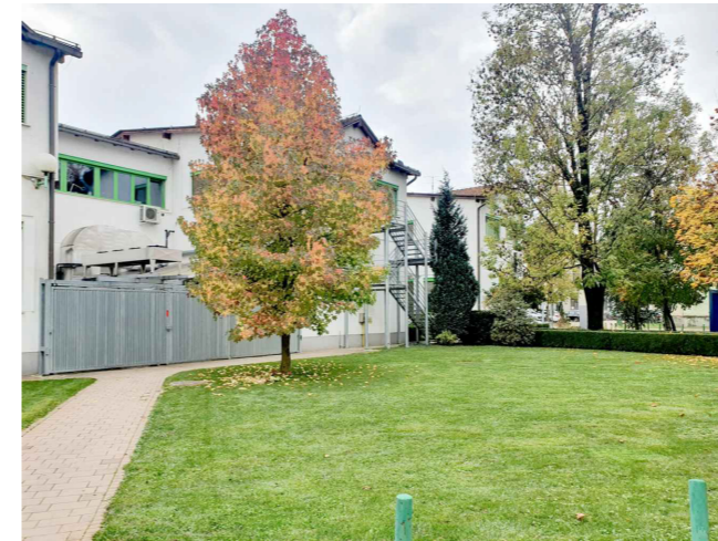
3 obstoječi park pred objektom IMI
